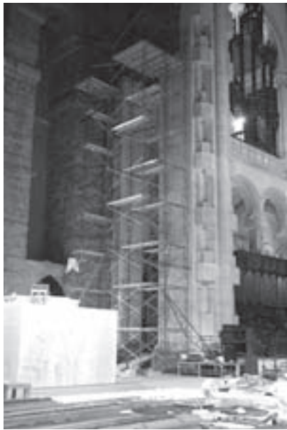
Scaffolding, St. John the Divine
