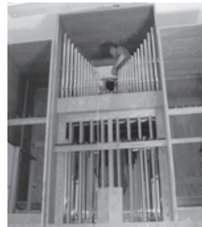
Pipes being removed from the University of Iowa's Schlicker organ (Photo by William Dickinson)
