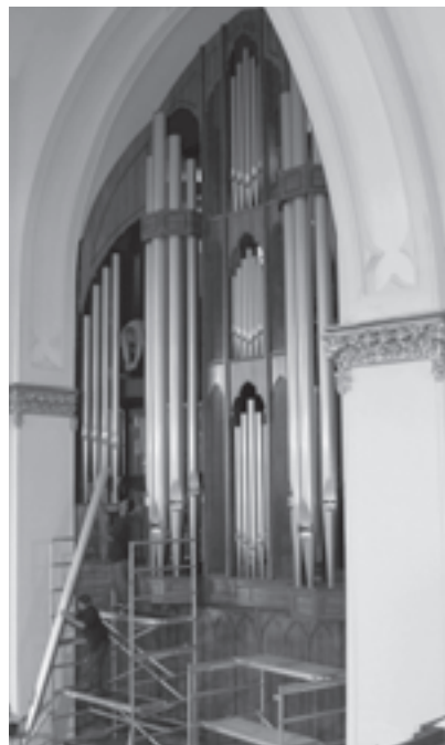
Installing façade pipes (photo credit Patty Conley)
