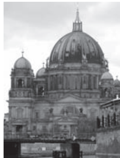
The Berliner Dom from the canal (photo: Jay Zoller)
