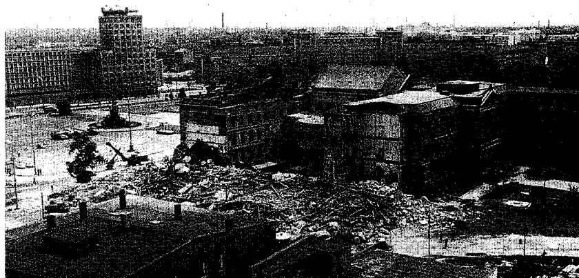
St. Paul's Church on May 30, 1968 a few hours after the detonation (photo: Bernhard Richter, Leipzig)
