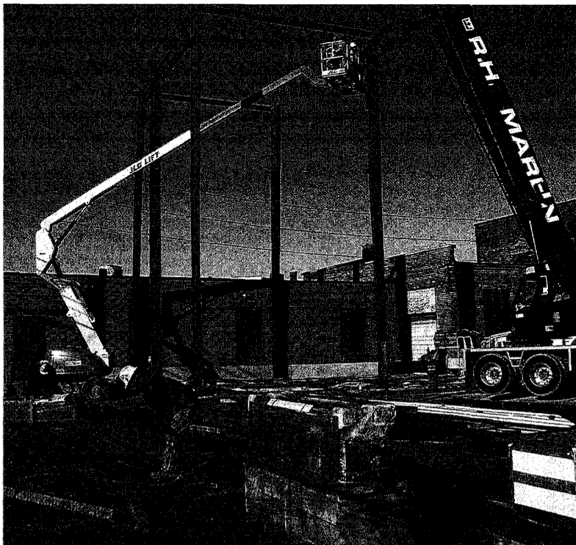
Goulding & Wood, Inc. new assembly room under construction
