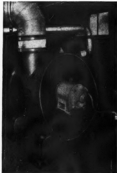
Five HP three stage, two pressure Orgoblo supplying wind at 4 1/2 and 6 inch pressures.
