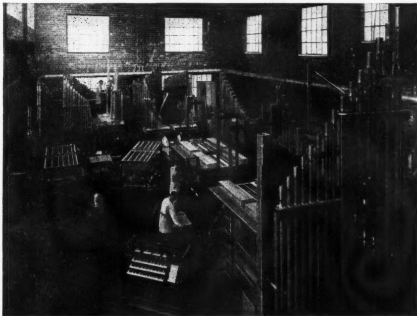
THE ASSEMBLY ROOM IN THE PRESENT KILGEN FACTORY.
