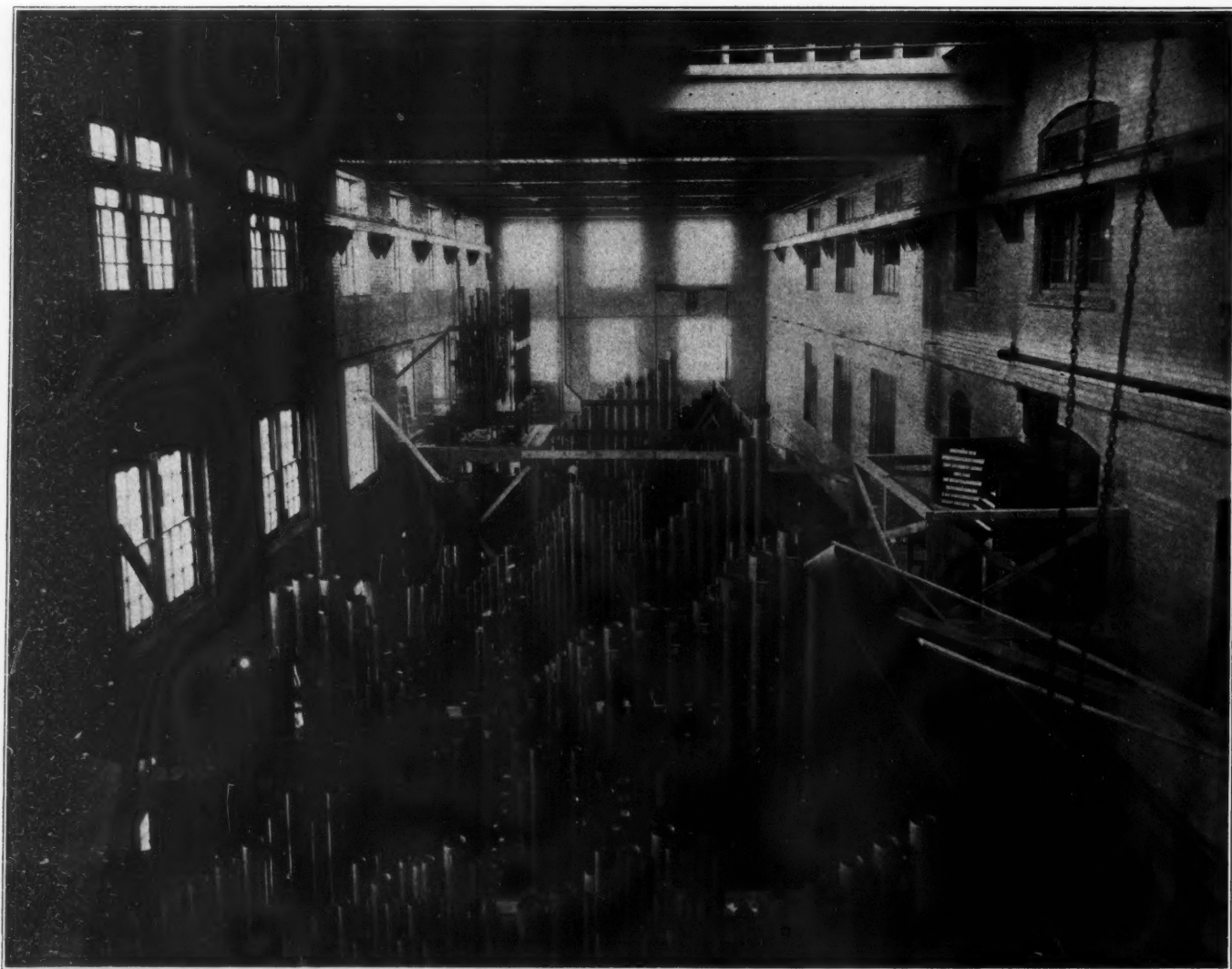
Parts of four sections of the Organ (three other sections not shown) with Console in testing position. Each expression chamber is a room with masonry walls, sound insulated.
