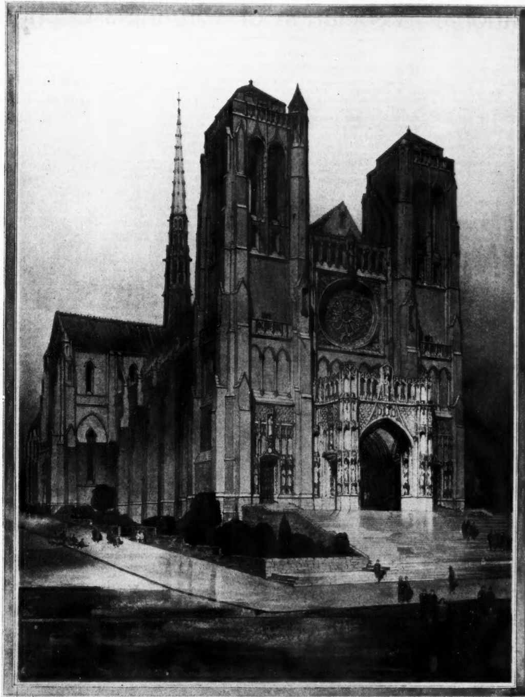
Lewis P. Hobart, Architect; Cram & Ferguson, Consulting Architects
