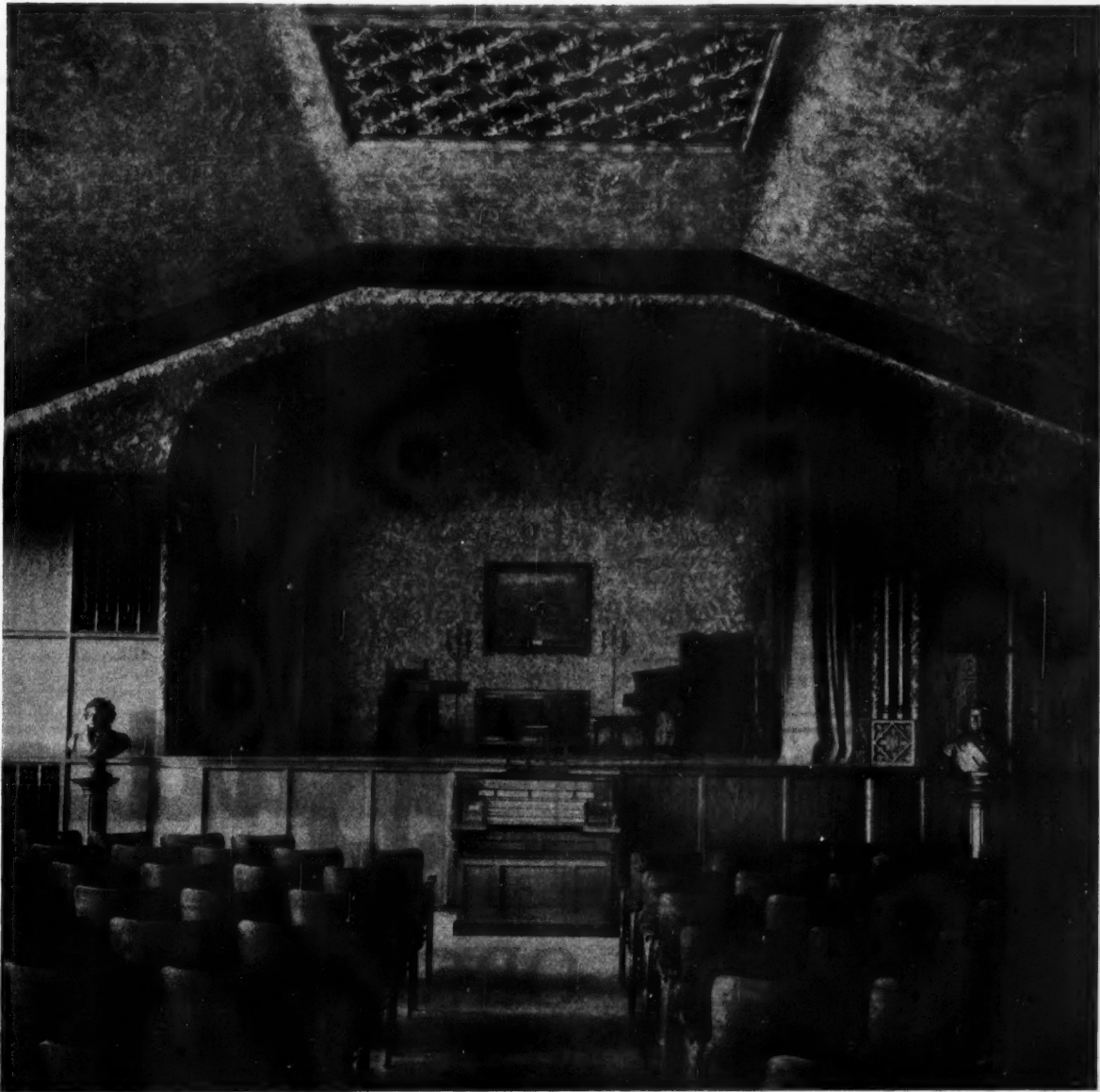
INTERESTING WELTE REPRODUCING ORGAN INSTALLATION RECENTLY COMPLETED IN THE WAGNALLS MEMORIAL BUILDING, LITHOPOLIS, OHIO. DEDICATED MAY 31, 1925
