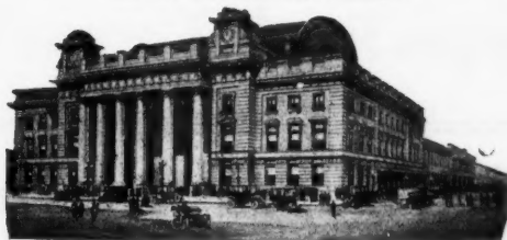
Chicago Passenger Terminal
