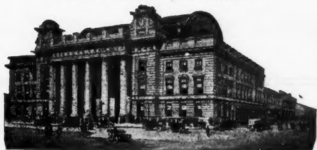
Chicago Passenger Terminal
