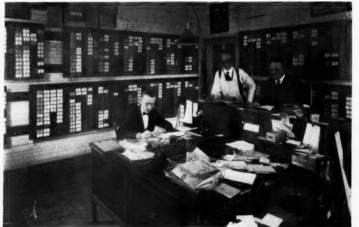
The drafting room sends out instructions on what to do. This is the production department which tells when to do it and what to do next. By means of the boards which cover the four walls the progress of the different parts of any organ are watched and followed until everything is ready, when space is assigned on the floor of the erection shop and these parts brought together and set up complete. Records of raw materials are also kept here, and stocks are kept up in cooperation with the purchasing department which is located in the next office.
