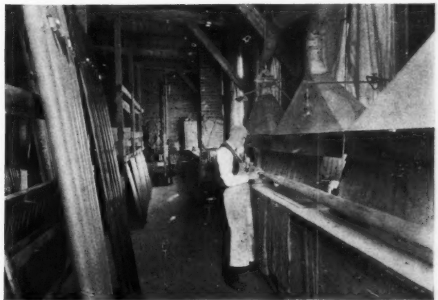
In this room the front pipes are decorated.
