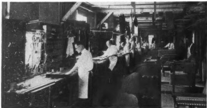
In this department the consoles are set up. The console case in the foreground is for a Luminous Stop Console. It is small and compact, occupying, without the pedal board, no more floor space than an upright piano.
