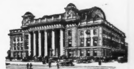
Chicago Passenger Terminal
