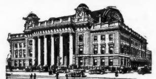
Chicago Passenger Terminal
