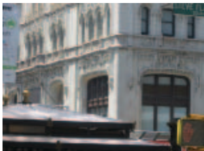
Woolworth Building, street-level detail
