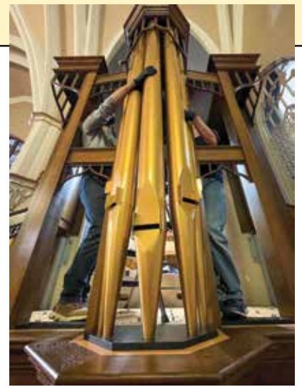
Façade pipe installation
