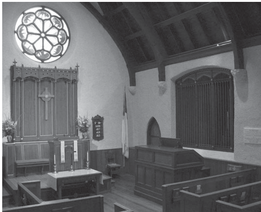
The chancel grille is 80% openwork to permit unencumbered pipe speech.
