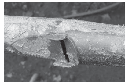
Façade pipes required special treatment in order to remove old layers of paint
