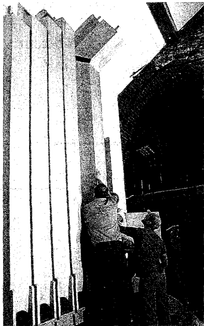
Installing bass pipes
