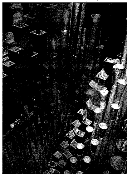
Hook Great pipework
