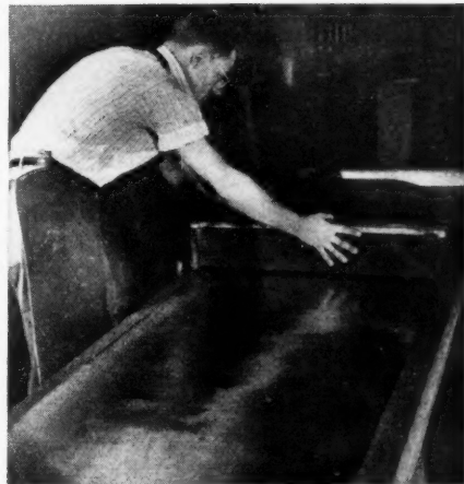
▶ THE MOLTEN METAL HAS BECOME A SHEET ON THE CASTING BED. IT IS READY FOR THE PIPE MAKER.
